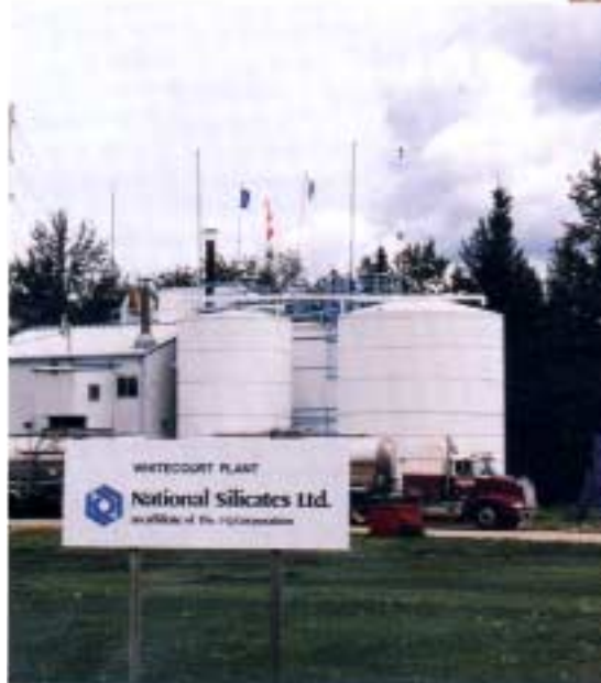
National Silicates Ltd. operates a satellite plant at Whitecourt.
